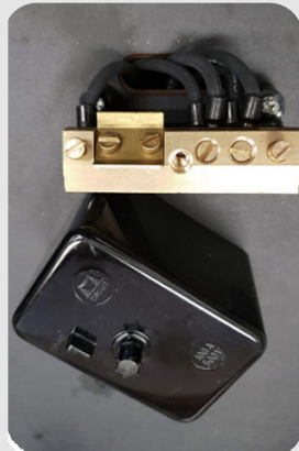
Meter Neutral Link
